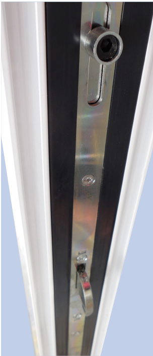
View of lower hook bolt and cam
